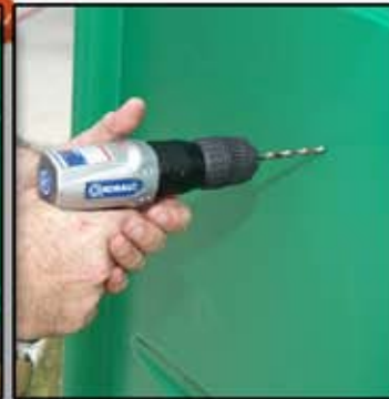
4 Locate holes on the outside of the toilet to align with the holes in the Wash Unit. Drill holes from outside of toilet into wash unit.
