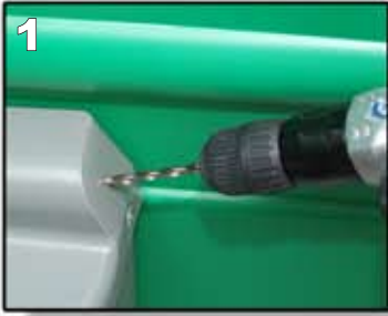
1 Drill 1/2" hole in toilet tank using molded indentation as a guide.
