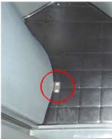
6 Push tank against inside wall. Mark and drill holes in floor for bracket. Attach bracket to floor with rivets.
